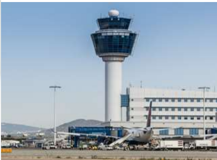
ATHENS INTERNATIONAL AIRPORT
